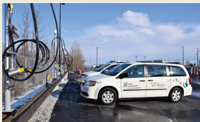
Natural gas vehicle re-fueling station using biogas
