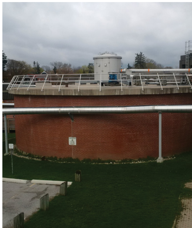
Anaerobic digester at City of Barrie Wastewater Treatment Facility. Source: City of Barrie.
