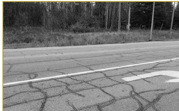
Six-year-old highway with premature cracks, in Coldwater, Ontario.
