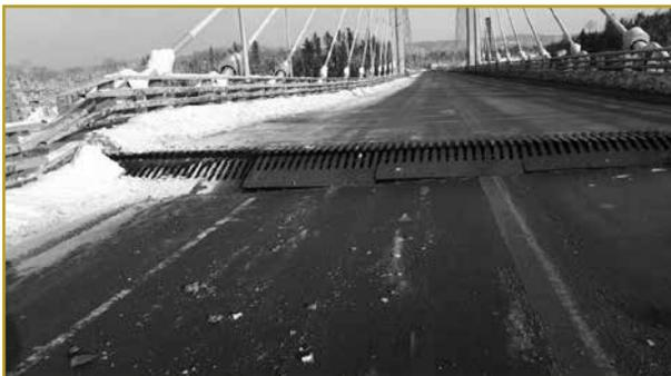
The Nipigon River Bridge failed after one end rose by 60 cm.
